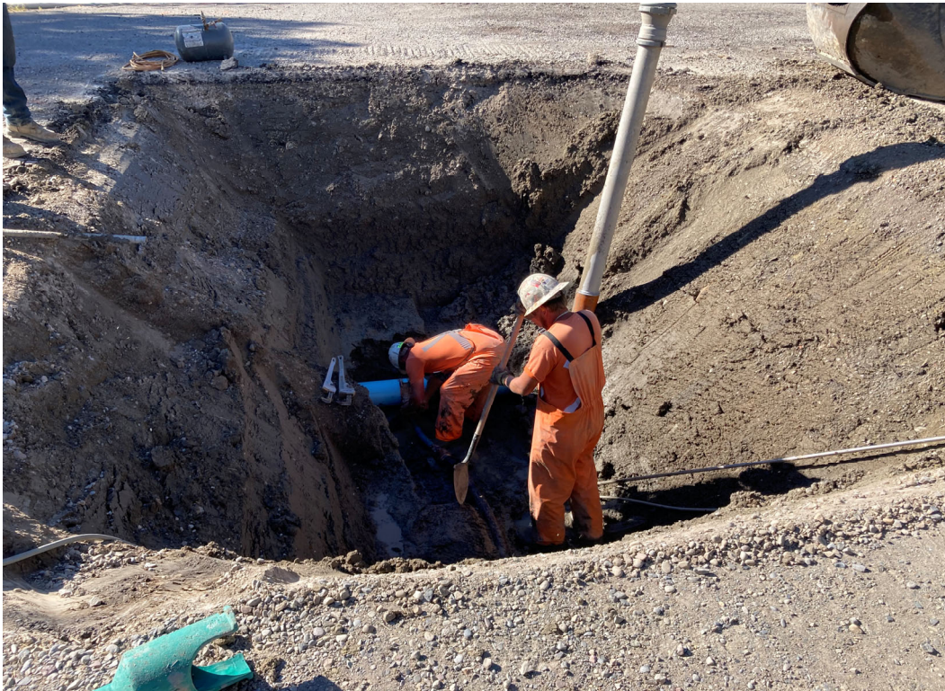
Picture 2: Valve Installation
