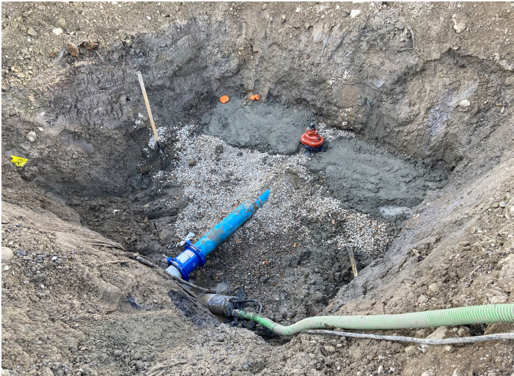
Picture 6: Valve Installation
