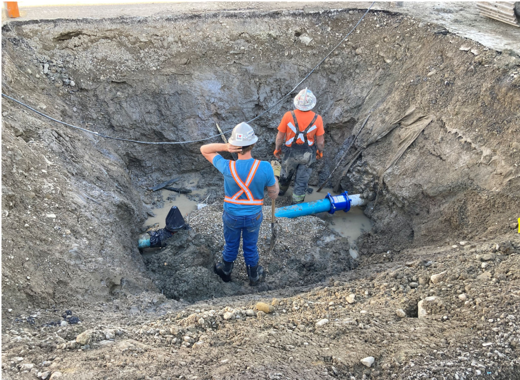
Picture 4: Leak Repair and Valve Replacement
