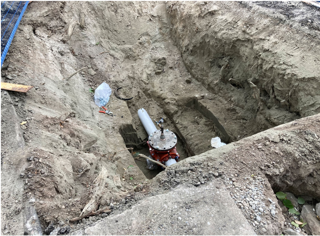
Picture 3: Valve Replacement
