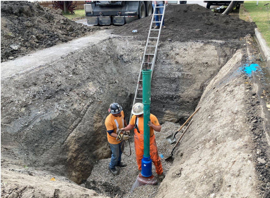
Picture 7: Valve installation
