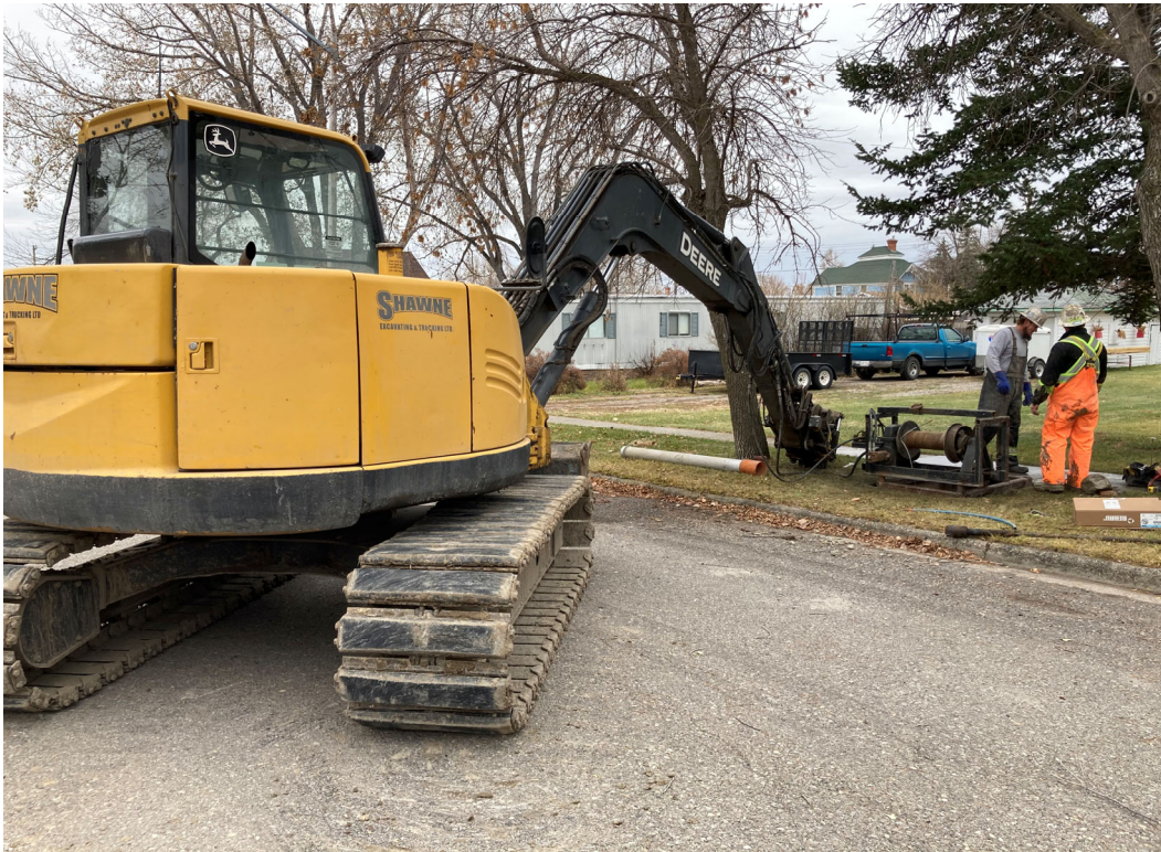
Picture 9: Curb Stop Replacement and Service Pull
