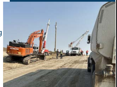
Range Road 263 Grading and Utility Relocation
