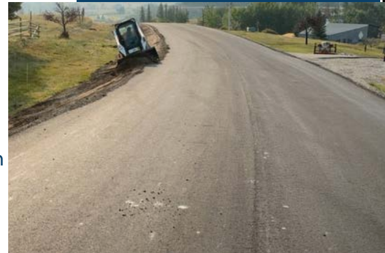
Moon River Drive Finishing Work
