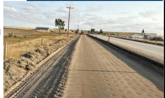
Range Road 263 Base work
