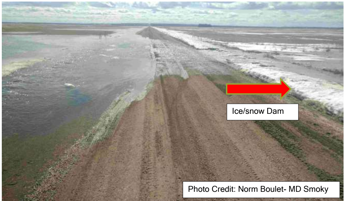
Picture 1. Ditch ice/snow dam create flooding on fields but also on road.
